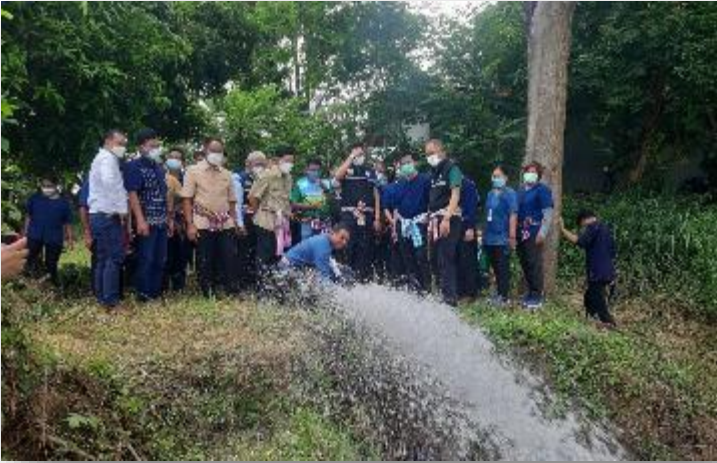
3. Cooperate with Community with project "Irrigation Piping" for local agriculture
